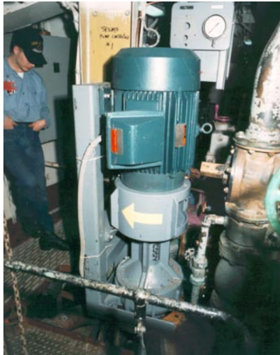
Figure 6. Eddy Pump installation in CVN 68.
